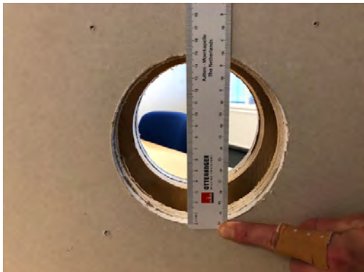
fig 1- Core hole trough the wall
