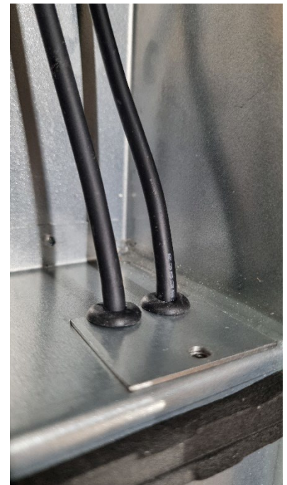
Slide the metal plate back into the opening of the rubber rings. Screw tight.
