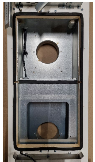
Clean both compartments with a vacuum cleaner. Check the inlet and outlet pipes for leaves etc.
