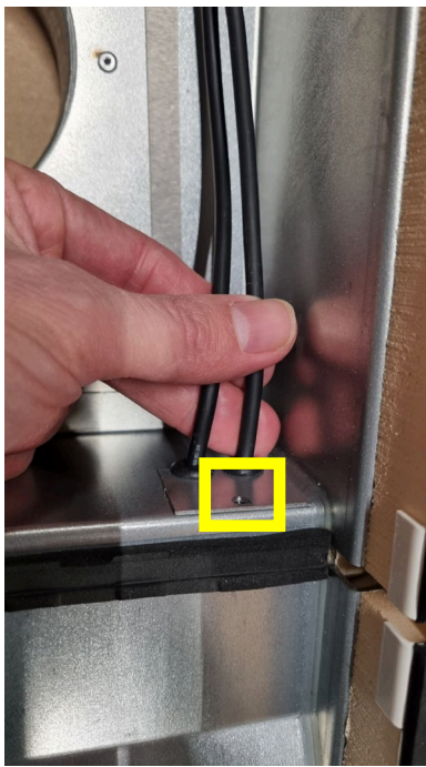
Loosen the screw of the small cable plate
