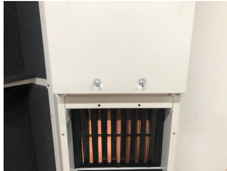
Figure 3 Top cover thumb screw
