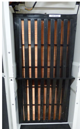
Figure 5 – Heat exchanger ready to be removed
