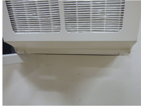
Figure 2 – Filter inserted into hooks on unibody
