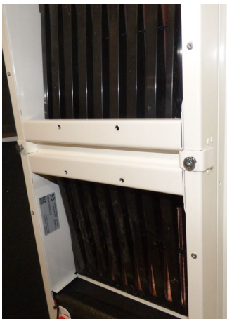
Figure 4 - Fresh-r middle bar separator
