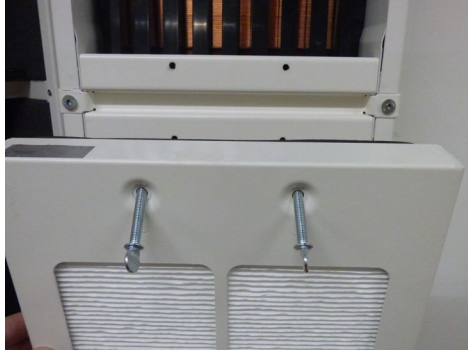
Figure 1 - Filter thumb screws
