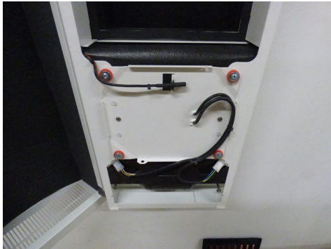
Figure 3 fan module as installed
